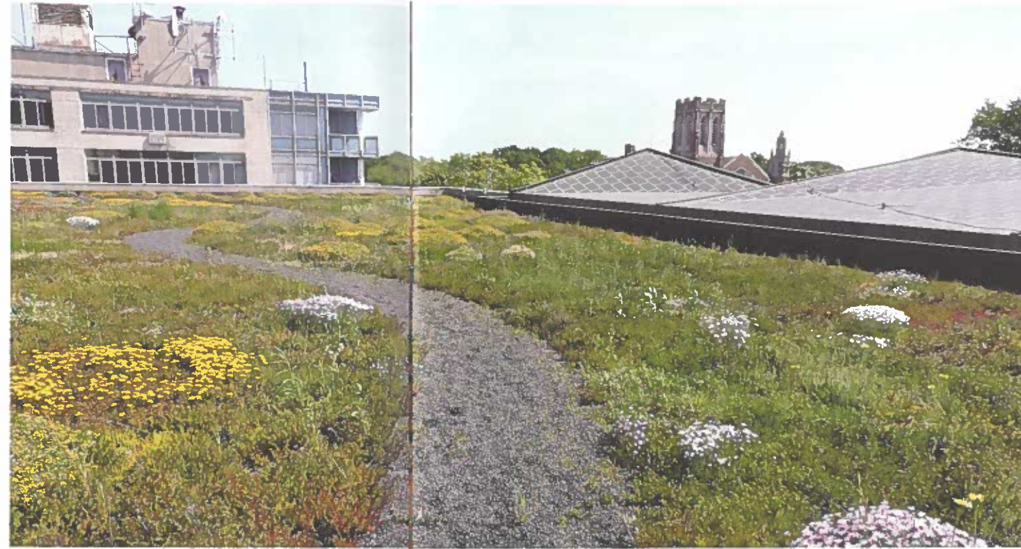
The Main Library's green roof in May 2016.
